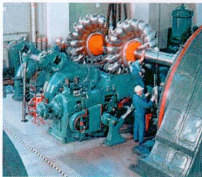
Impulse turbine being installed
