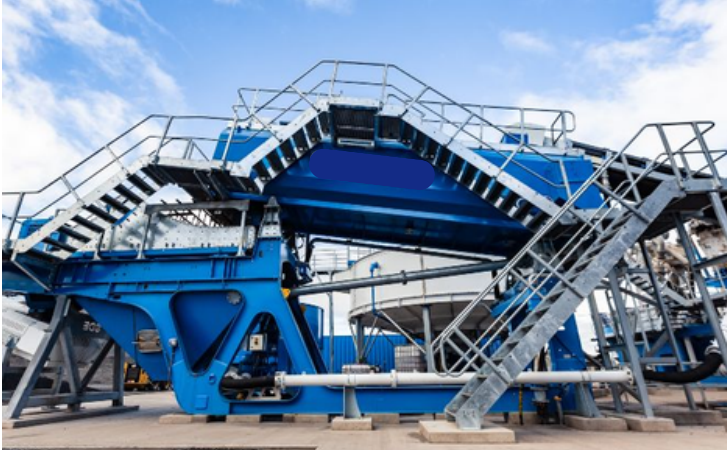
Scrubbing & Classification system
