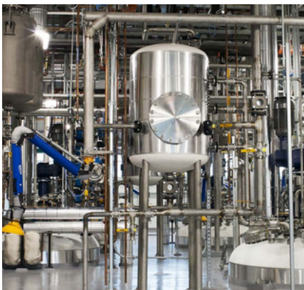
Chemical Filtration Equipment
