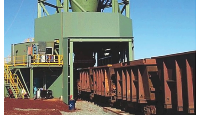
Loading ,Unloading & Train Station
