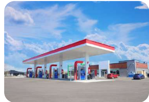
Complete system for petrol station
